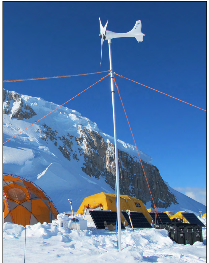
New solar and wind power system used for Badger-Eclipse drilling in Denali National Park. Photo: Mike Waszkiewicz
