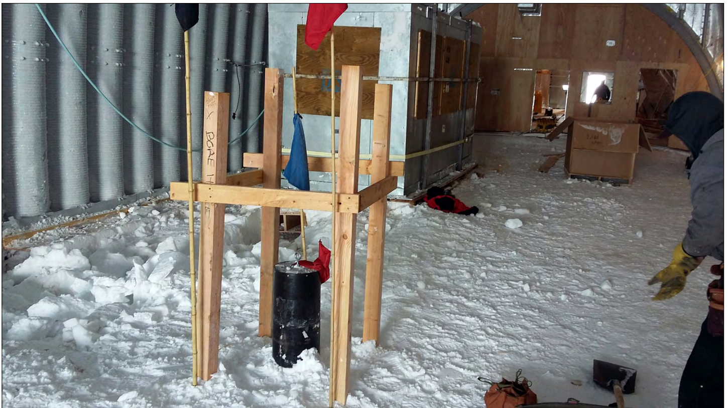
The borehole casing extension at WAIS Divide, Antarctica. Credit: Jim Koehler
