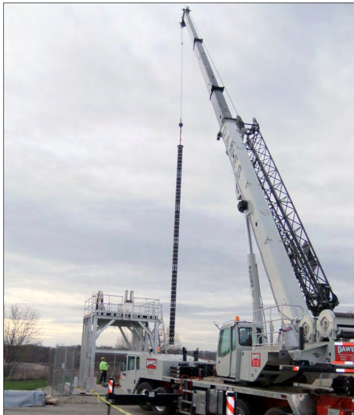
Preparing the temporary ice well at PSL for the North American Test of the ASIG Drill. Credit: Chris Gibson
