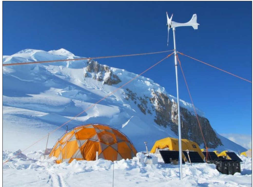
Eclipse Drill renewable energy system 1 kW solar array and 600 W wind turbine
