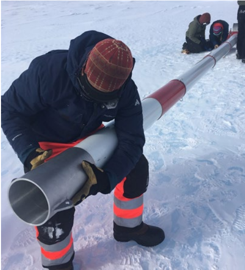
Figure 9-7: Tent pulley anchor tube seats on top of the spacer tube.
