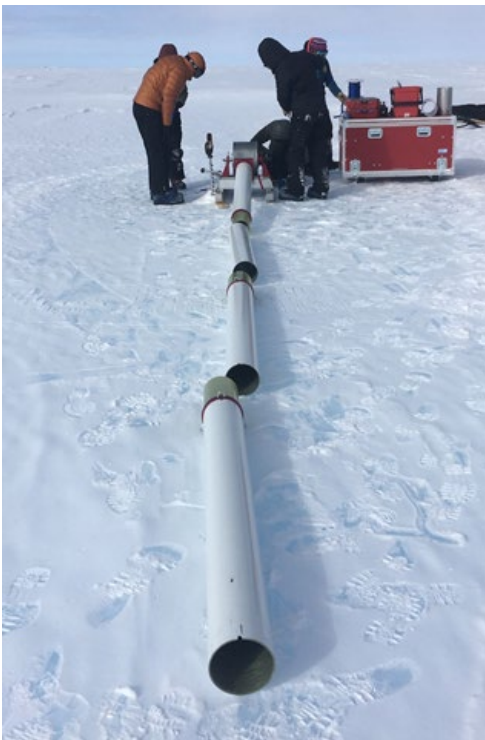
Figure 9-5: Tower sections with tower tube couplings.
