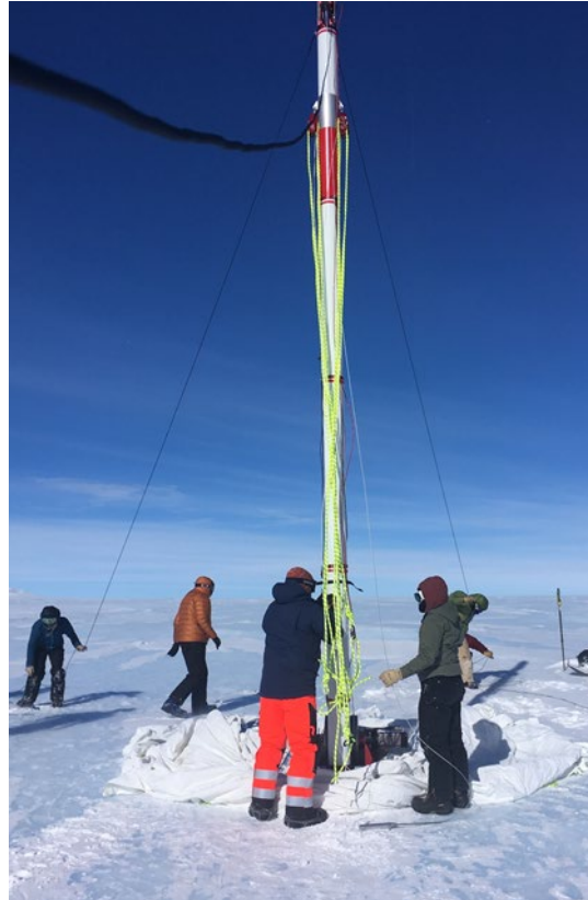
Figure 12-1: Raising the drill tower with drill tent body and rigging. Note: the old tube tower is shown in this picture.
