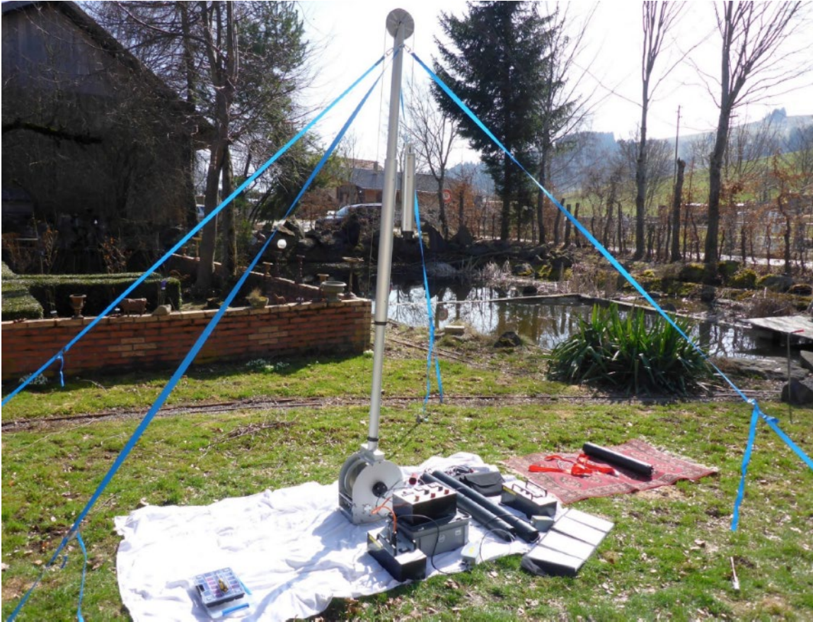
Figure 7: Ready for drilling
