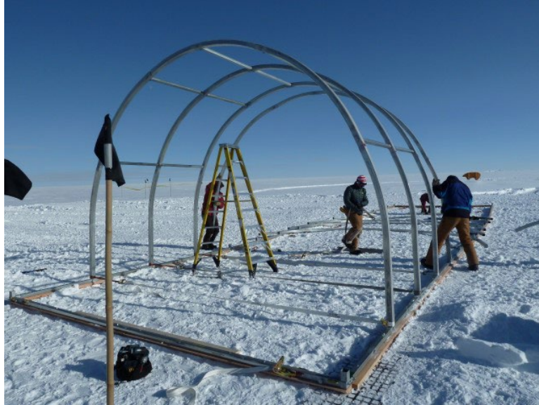
Figure 5. Tent frame being assembled off the end of the trench and on the Geoblock footing tails. Note: this picture is of the Foro 1650 tent, but the assembly process is the same for Foro 3000.
