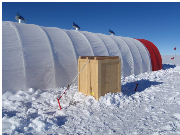
Figure 46: Cover over the slot ventilation fan.
