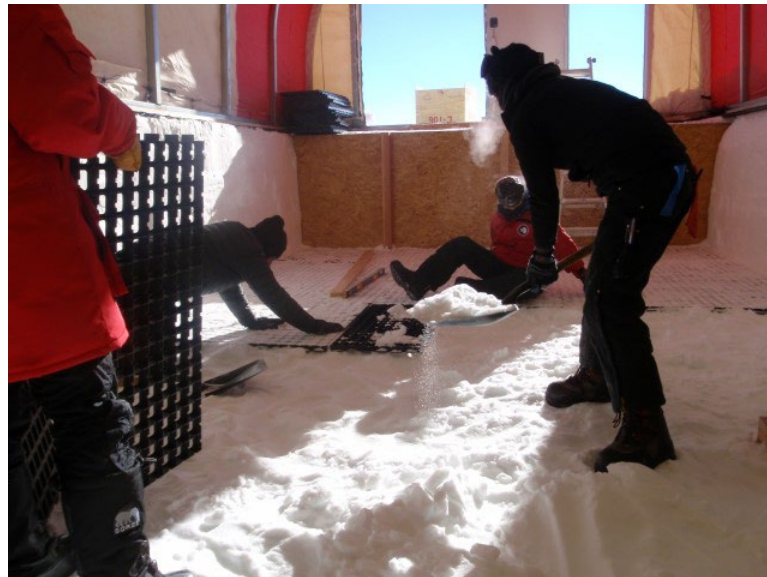
Figure 10. Installing the Geoblock flooring.
