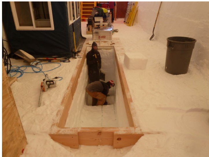
Figure 9. Slot excavation after the winch footing has been installed. Note, the picture is of assembly of the Foro 1650 system, but the process is the same for Foro 3000.
