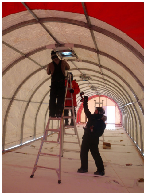
Figure 8. Installing the roof vent fans. Note: this picture is of the Foro 1650 tent, but the assembly process is the same for Foro 3000.
