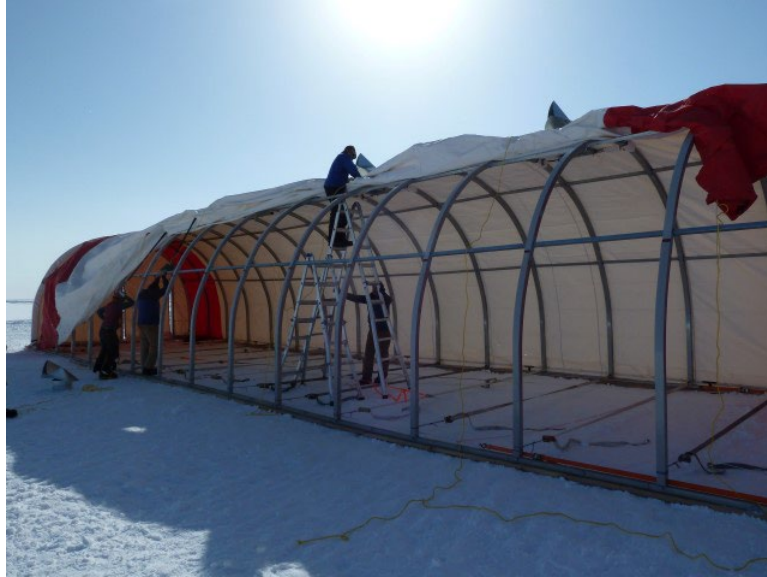
Figure 7. Installing the roof vents. Note: this picture is of the Foro 1650 tent, but the assembly process is the same for Foro 3000.
