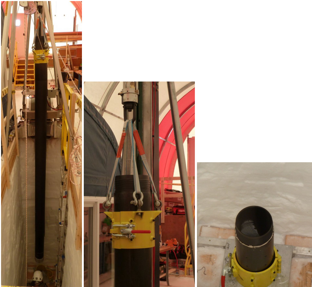
Figure 42: Installing a casing with threaded connections. Left; section of casing being lowered with the drill winch. Center; upper casing clamp. Right; lower casing clamp.
