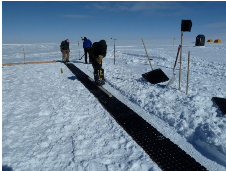
Figure 3. Installing the Geoblock tent footing
