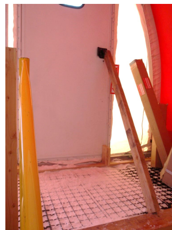
Figure 47: Bracing at the bottom and mid-point of the entry door.
