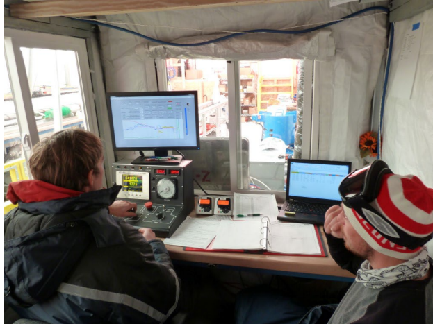
Figure 15. Drill control interface inside the control room tent. Note: This picture is from the Foro 1650 system, with the Foro 3000 system being similar.
