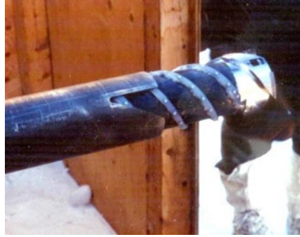
Figure 43. Extracting the Core Barrel
