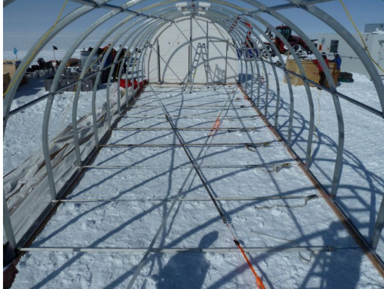
Figure 7. Assembled tent frame with straps to keep the base from spreading.
