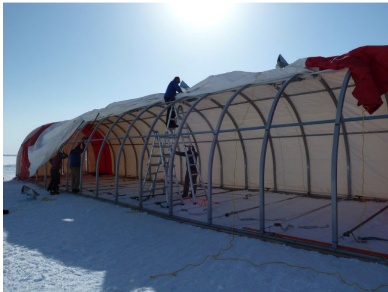
Figure 8. Installing the roof vents
