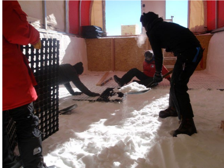
Figure 5. Installing the Geoblock flooring.
