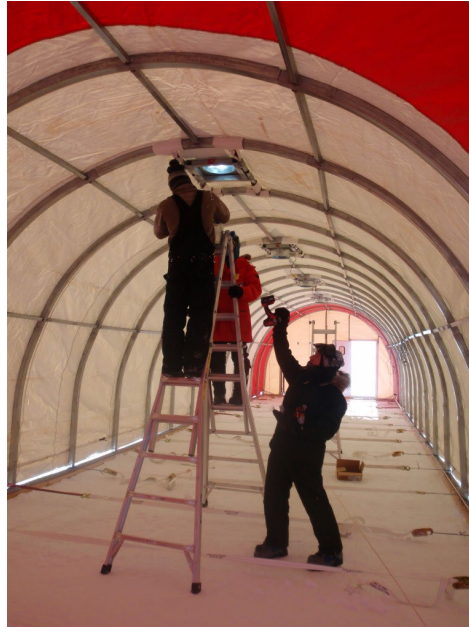
Figure 9. Installing the roof vent fans
