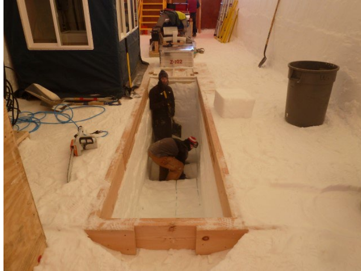
Figure 10. Slot excavation after the winch footing has been installed.
