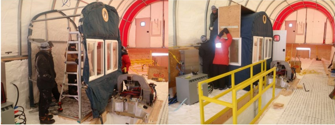
Figure 12. Left - Control Room assembly. Right - ERV system mount being installed.
