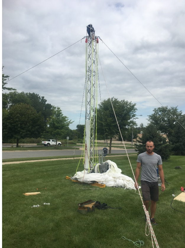
Figure 12: Secure 4 guy lines at 20' from bore hole with anchors appropriate for surface conditions.
