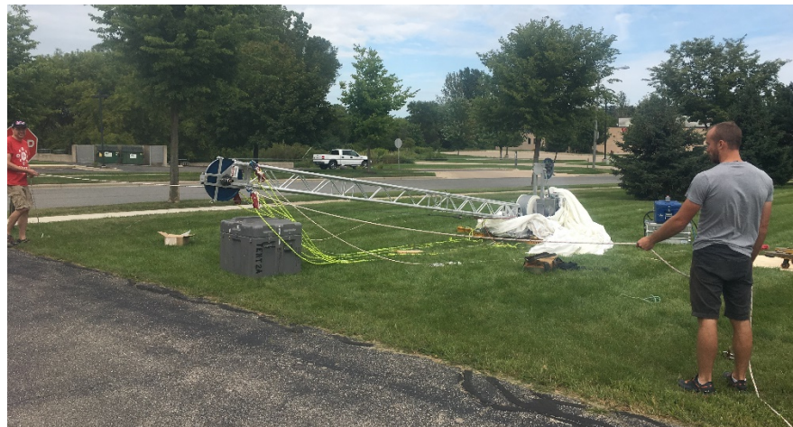
Figure 11: Tower Lifting. Two people stabilize tower with front guy lines.
