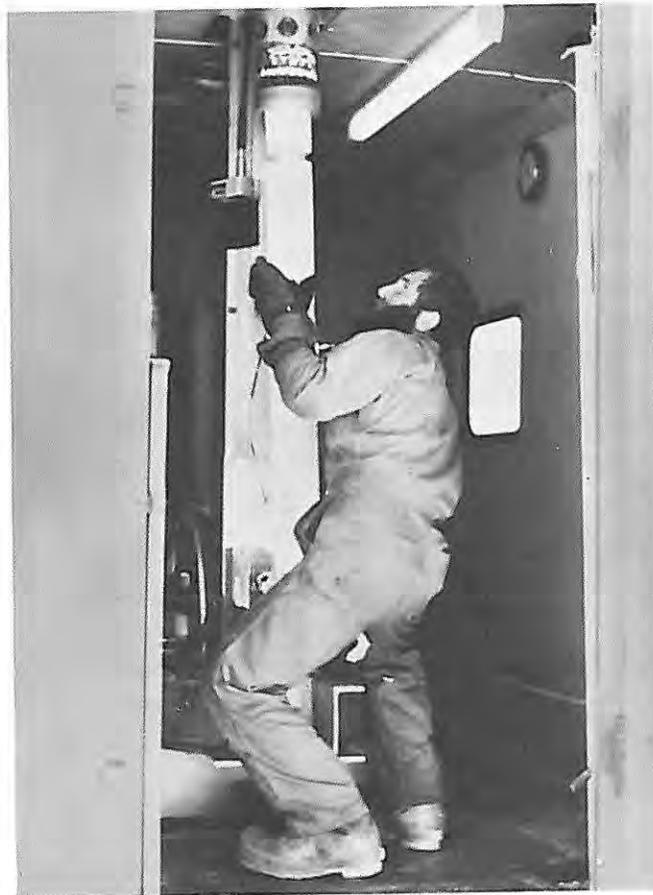
**Figure 8.** An ice core being removed from the thermal drill.
