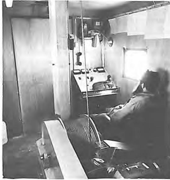
**Figure 5.** Ice drill in operation, showing the winch, control console and operator.
