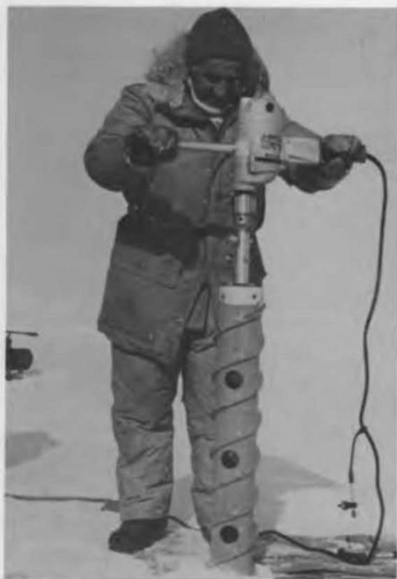
Figure 15. Prototype Rand auger with \frac{1}{4} -inch electric drive.
