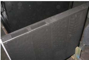
**Figure 15 – Typical Tray Air Inlet Area, and Edge Openings For Charcoal Refill**
