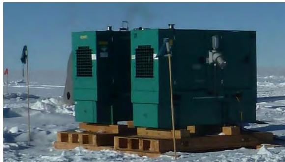
50 kW generators used for the SPICE Core project
