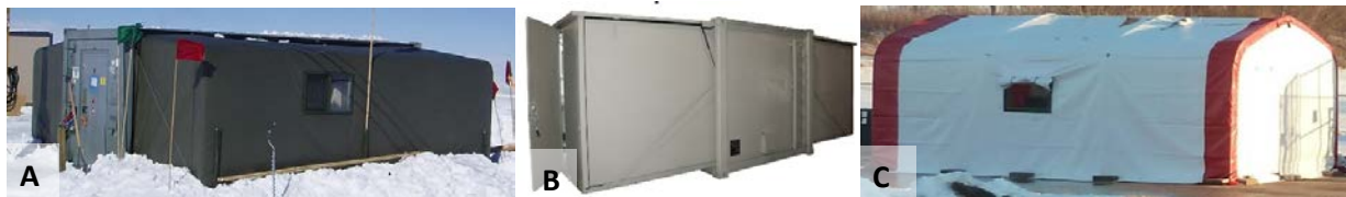
Figure 6: Mobile shop options. A – 20' expandable container (MECC), B – 10' expandable container (Bicon), C – tent
