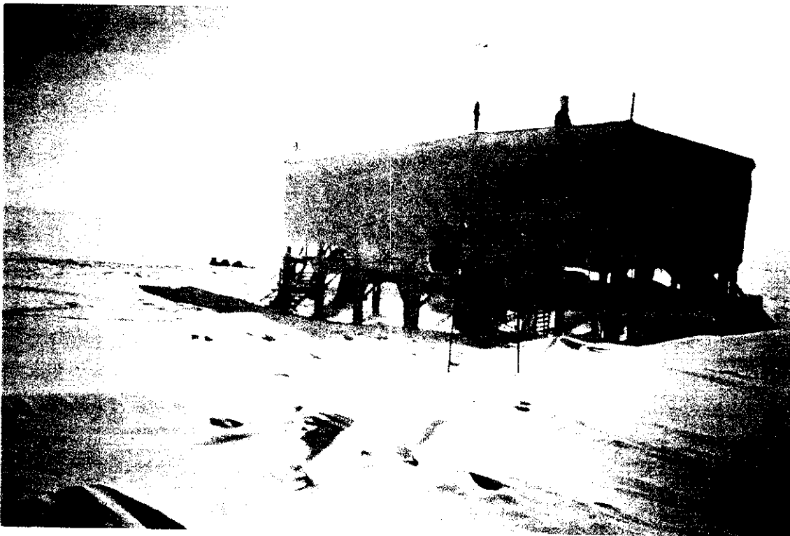
By 1993, the floor of the big house is 4' to 5' above the surrounding grade. Scouring was hampered by a utilidore extending from the building. It is expected that drifting will increase dramatically when the surrounding grade reaches the base of the walls.
