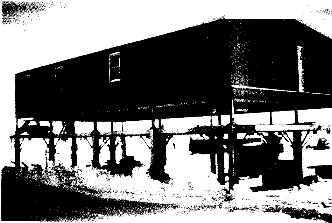
Based on a CRREL foundation design to permit scouring, this stress skin panel building known as the big house, sits on piling approximately 10' above grade and was completed in 1990.
