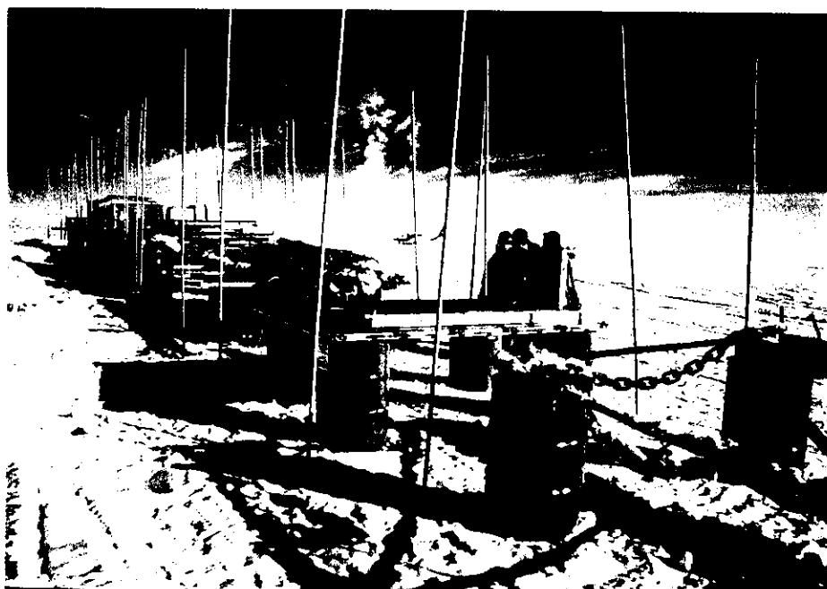
At the end of the season, winter-over pallets are raised on berms and/or drums to minimize burial during winter-over.
