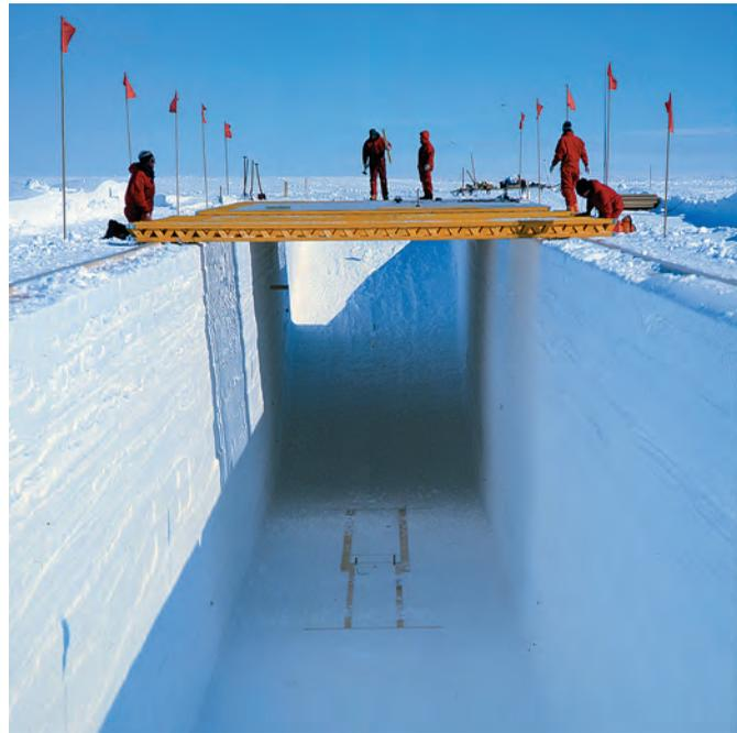
**Fig. 14:** Drill and science trench under construction: After the trench was excavated, it was covered with a wooden roof. The roof rests on wooden beams on top of compacted snow (see Fig. 13). On the ground of the six metres deep trench one recognizes the wooden foundation for the winch and the drill tower. (Photo H. Oerter, January 2001).
