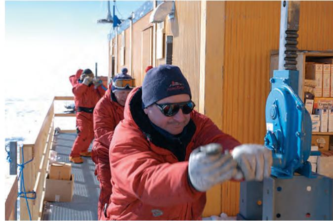
**Fig. 11:** Jacking up of the platform of Kohnen Station by winches mounted on top of the extended pillars. Each synchronous turn of the winches lifts the platform by three millimetres. (Photo H. Oerter, 18.01.2008).
