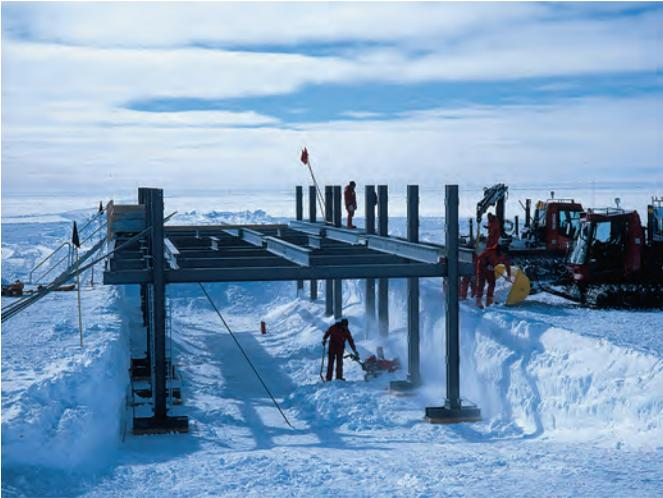
**Fig. 10:** Kohnen Station under construction. The excavation for the 16 pillars and the steel platform was 2 m deep (cf. Fig. 9). Some of the footplates under the pillars are already covered with snow by means of a small snow blower. Later the whole excavation was filled completely with snow. (Photo H. Oerter, 06.01.2000).
