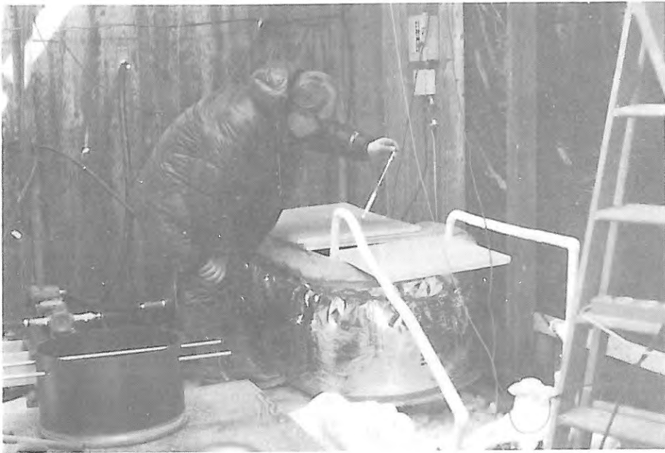
Fig. A33. Checking density in mixing tank.
