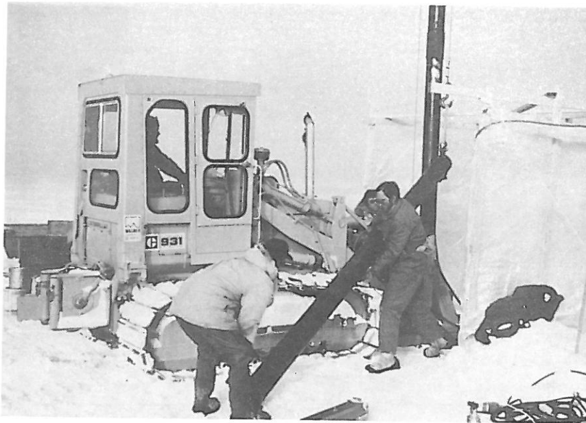
Fig. B-11. Casing being lifted into position.
