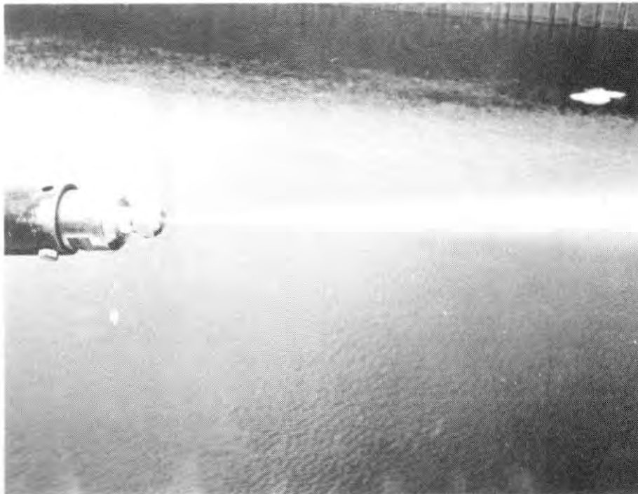
Figure 5. High pressure water jet used for cutting ice from lock walls.
