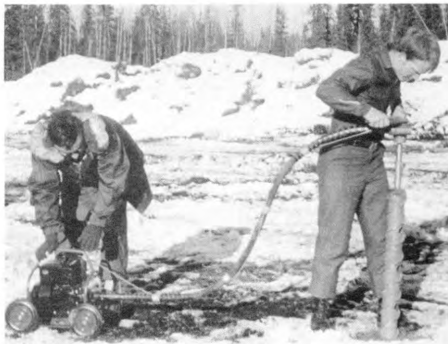
Figure A5. Coring auger with flexible drive cable and separate 5-hp engine on a dolly.
