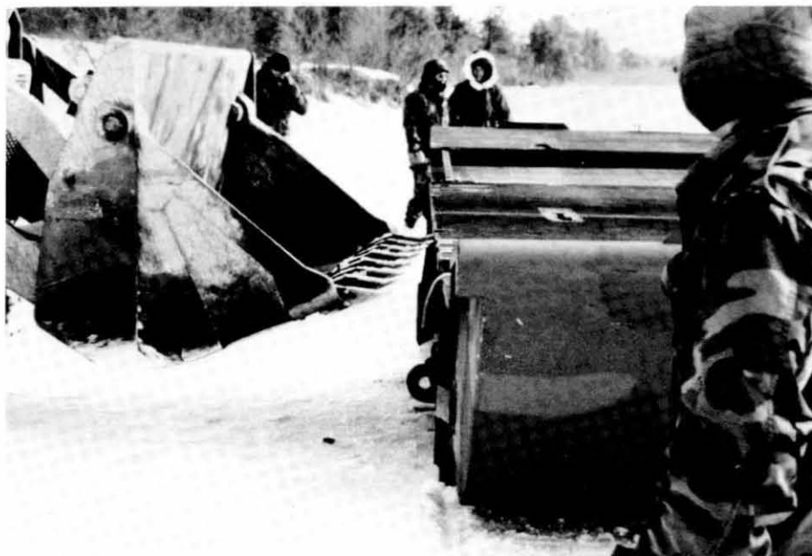
c. The bulldozer blade was used to carefully lift the bay to allow the bow ponton to swing into position.
