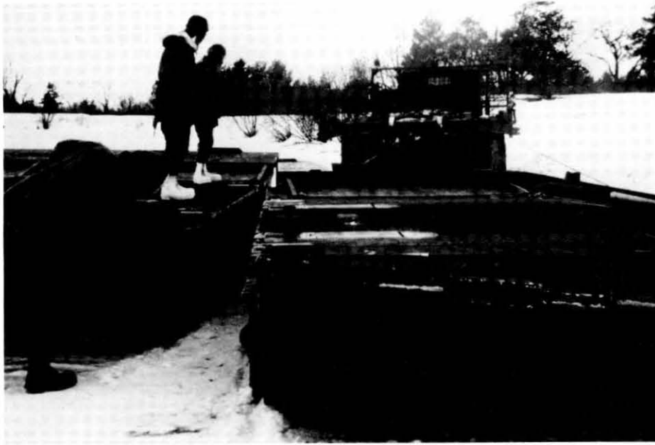
c. Once aligned, the ramp bay was moved sideways into position at the end of the interior sections.
