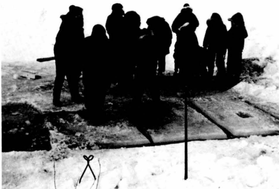
Figure 6. Ice cut into three sections, showing the lifting hole in the righthand block.
