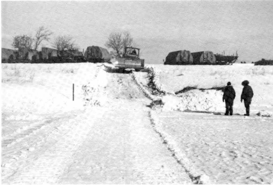
Figure 9. Bulldozer clearing the snow from the north side of the crossing lane at Alderwood Lake.
