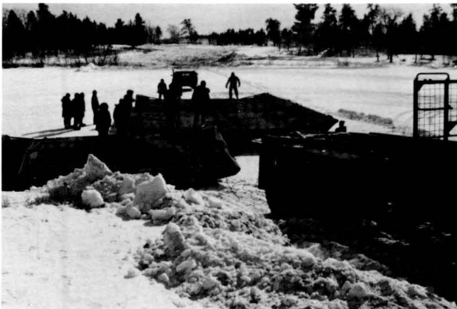
Figure 14. Deploying the ramp section.
