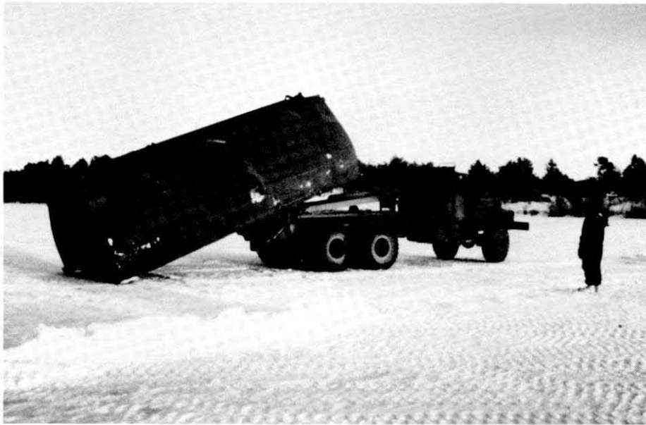
a. One end of the interior bay is slowly lowered off the truck to the ice.
