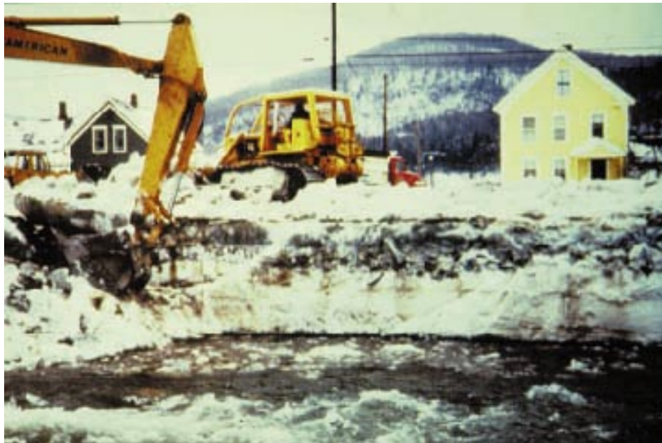
Figure 19. Breaching an ice jam in Hardwick, Vermont, using excavation equipment working from the shore and a bridge (bridge is not shown, but is just beyond the left edge of the photograph).
