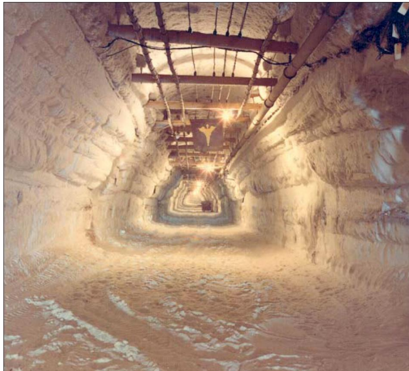
Fig. 1. Main 400-m-long access trench below the surface at Camp Century, 1964; more than a dozen, 150-m-long side trenches radiated out from the main trench ( Langway, 2008 )
