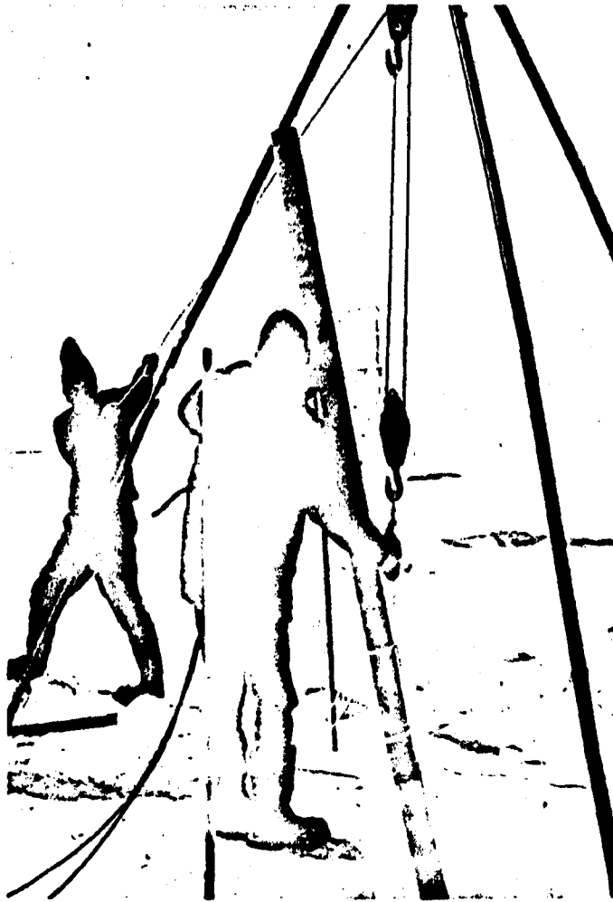
Fig. 3. Lowering the Probe in the 4.5 m Shaft; Thereupon, Oil Was Poured in, Filling the Cavity in and Above the Winding Reels.
