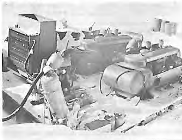
Figure 4. Air-to-air heat exchanger (left) and two 315-ft 3 /min compressors (right).
