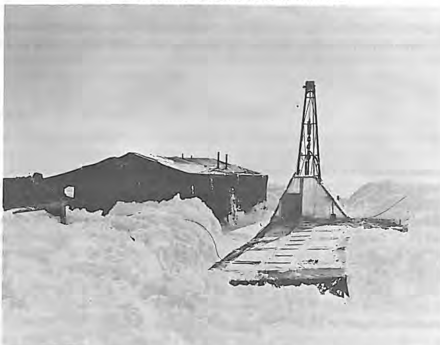
Figure 11. Rig and roof in place, compressor shelter on left, Greenland, 1957.
