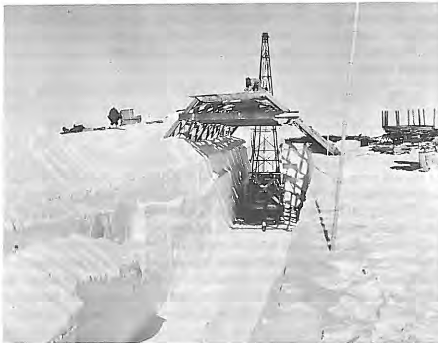
Figure 10. Trench excavated, rig in place and roof under construction, Site 2, 1956.
