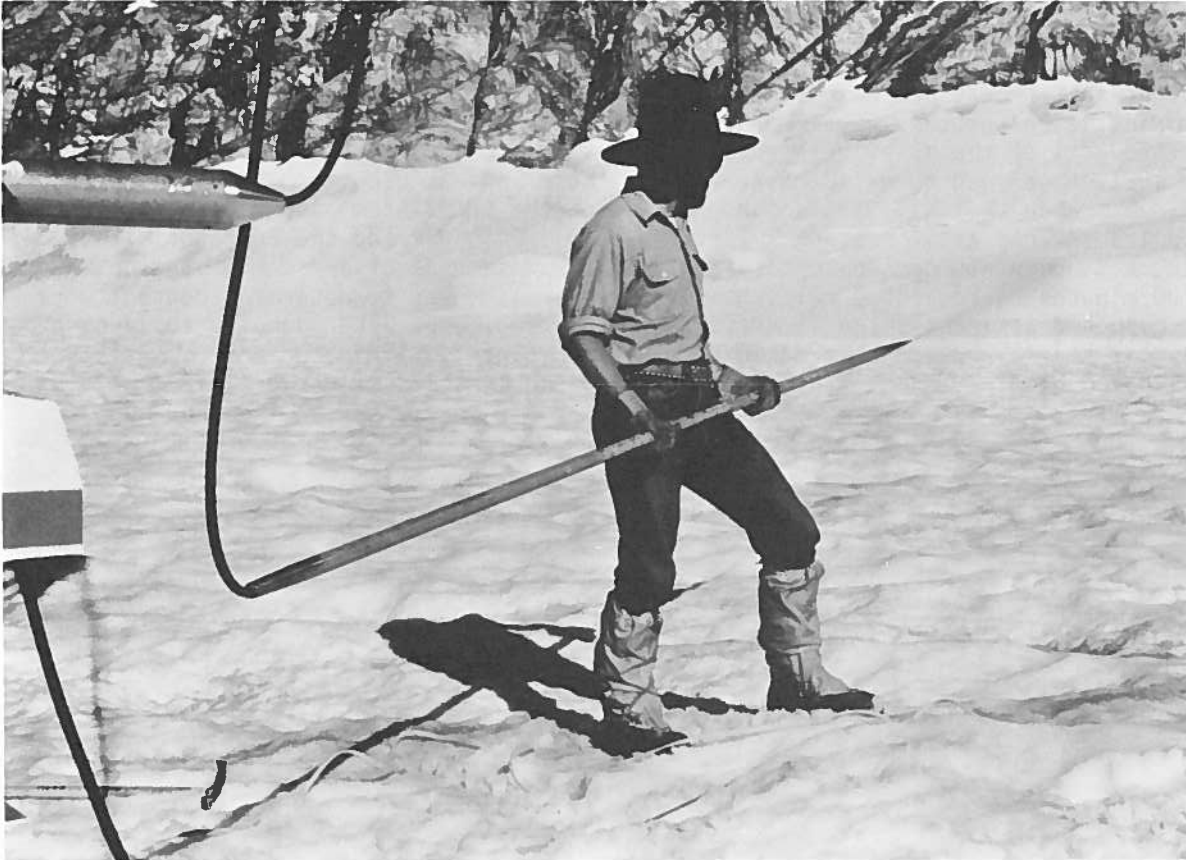
Figure 8. The hot-water drill stem.
