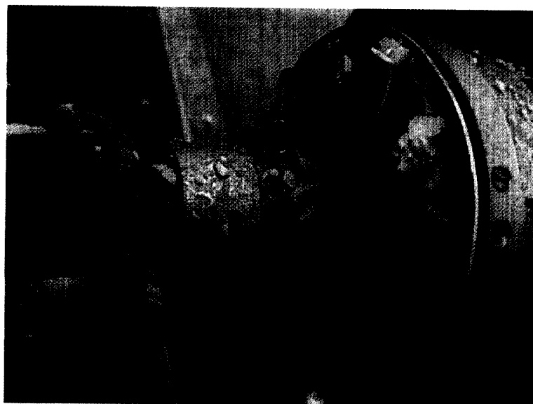
Fig. 5. Pump flap valve with big pieces of ice.
